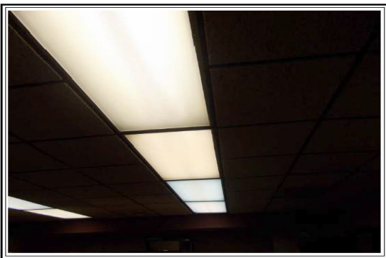
view of ceiling coverings and lighting fixtures
