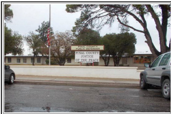
view of improvements across the street to the west
