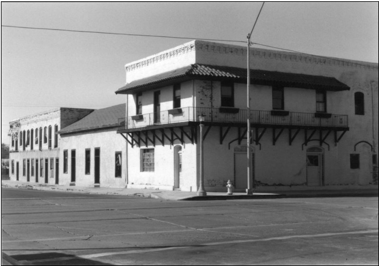
Figure 6. The Silver King Hotel in 1991 showing the rear adobe sections. Photo by Robert Stryker.
