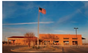
Florence Field Maintenance Shop CMAR
