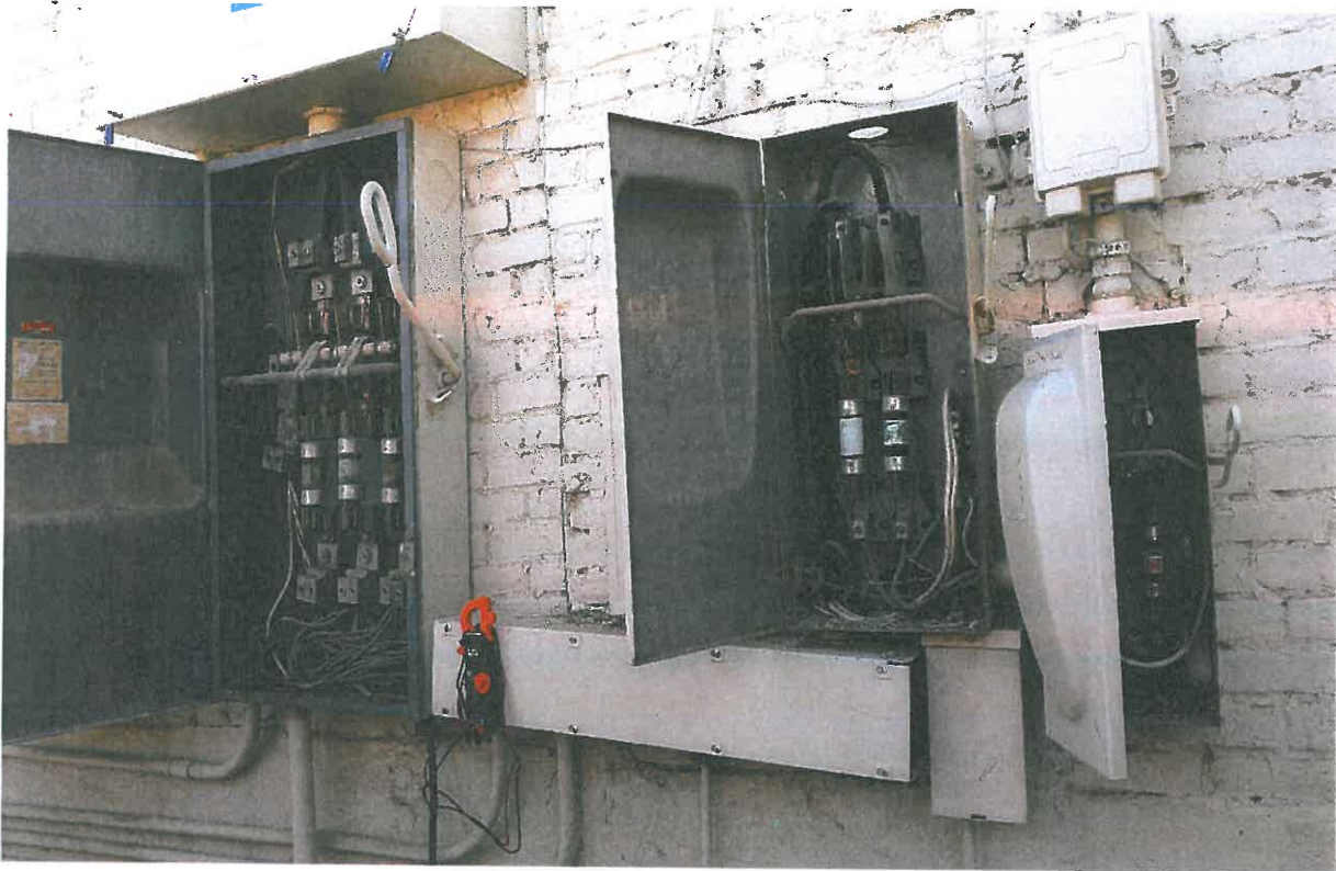
Electrical Service Box (Weather Head)
