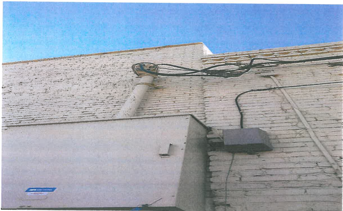
Electrical Service Box (Weather Head)
