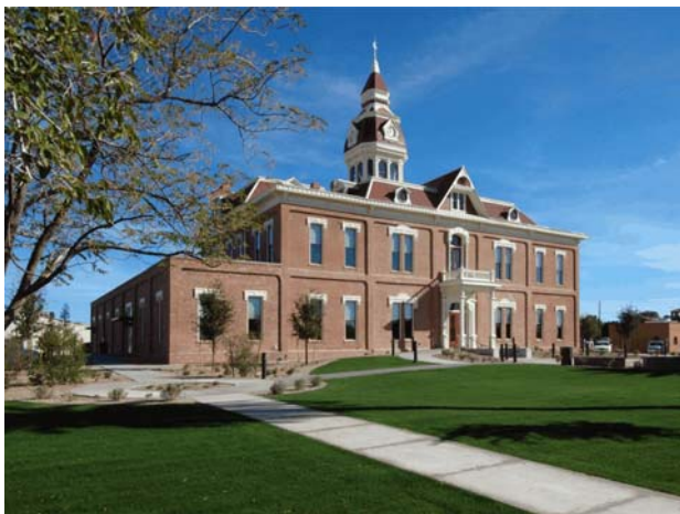
Pinal County Courthouse
