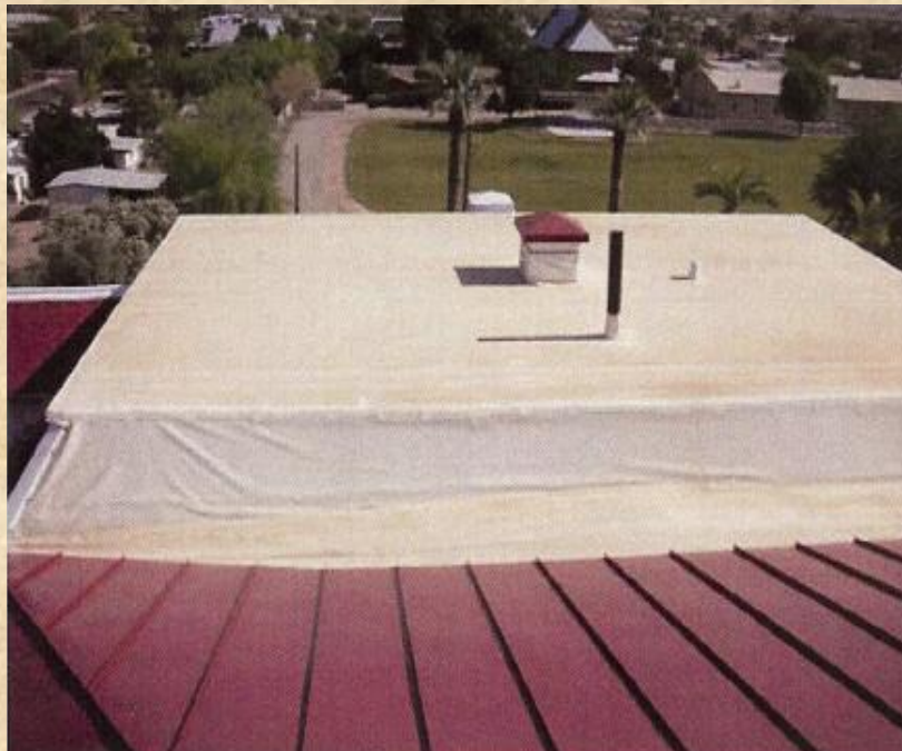
Recently installed membrane roofing and standing seam metal roofing above 1891 Courthouse
