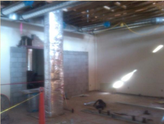
Infill of Masonry at Restrooms March 2012
