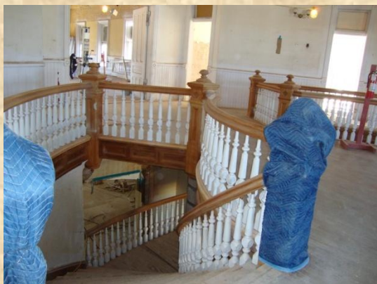
Lead paint removed from stairs.
