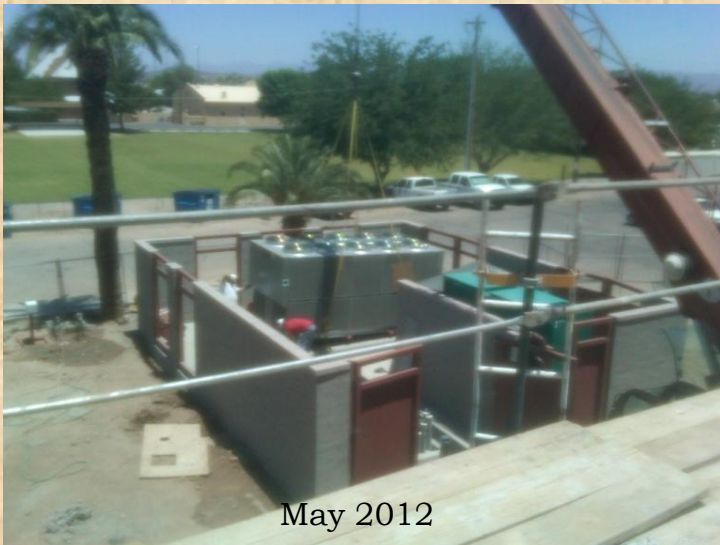
Setting equipment in Mechanical Yard
