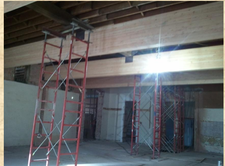
New Gluelam Beams installed – February 2012
