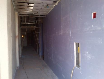
North hallway framed and sound board installed June 2012
