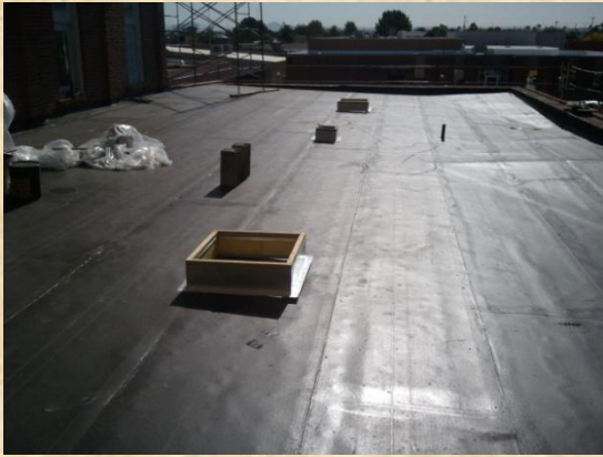
Base layer of roofing at south lower roof - April 2012
