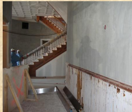
North hallway framed and sound board installed June 2012
