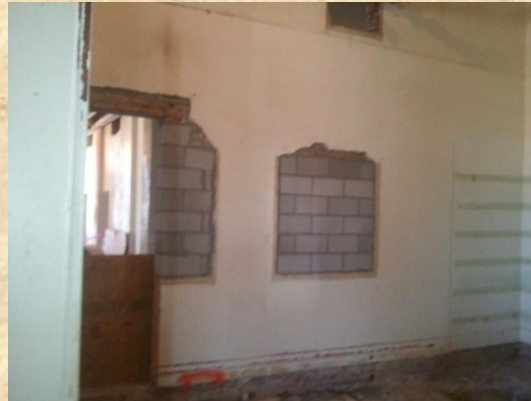
Lintel and Infill at Janitor Room March 2012
