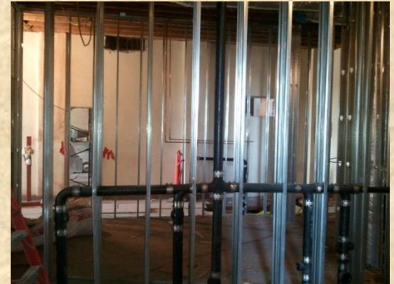
Plumbing rough-in at large 1 st Floor Restrooms April 2012
