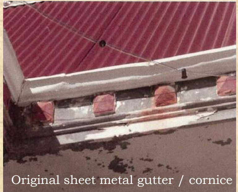
Original sheet metal cornice / dentils
