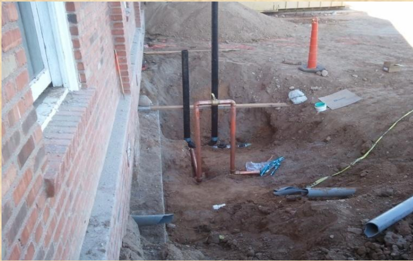
New Sewer tie-in and water connection February 2012
