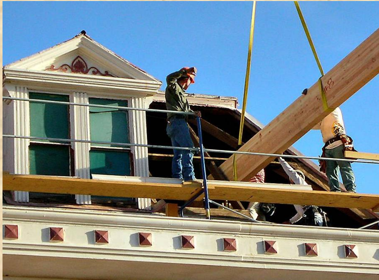
Installing support beams
