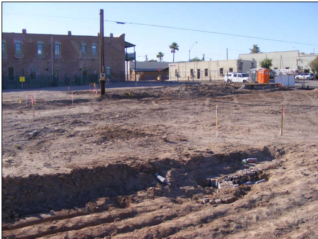
Photograph 1. Project area conditions at the start of construction. Feature 1 in Block 78 is in the foreground, and Block 79 and the Silver King Plaza is in the background, view to southeast.
