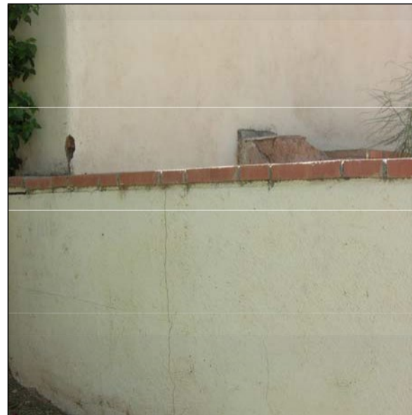
Stucco Wall with Brick Cap
